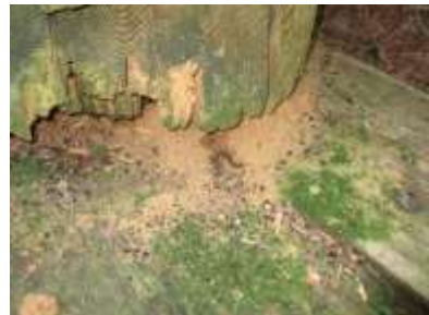
Note the fine sawdust around the base of the pole, indicative of insect activity.
