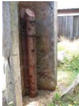
One type of support used for the outdoor totem poles.
