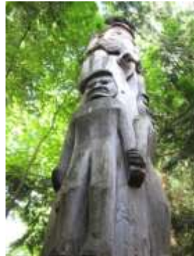
Notice the silvery hue to this weathered pole, indicative that the earlywood has been
